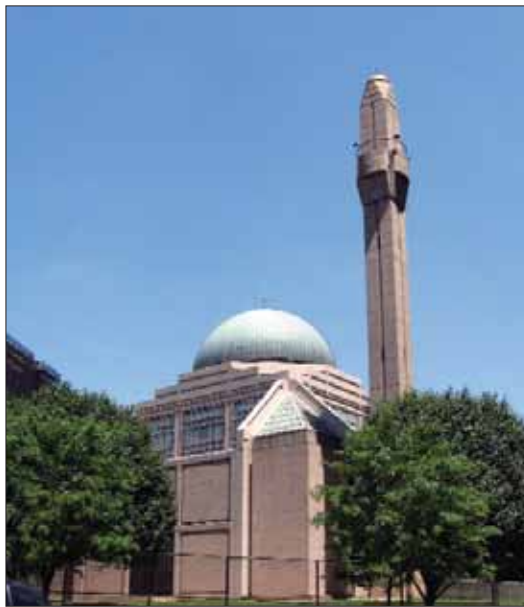
The Islamic Cultural Center on East 96th Street Photo: Jim Henderson
